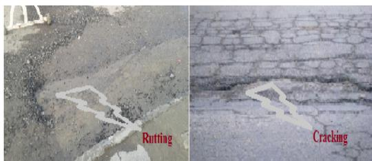
Fig. 1. Figure showing some pavement defects
